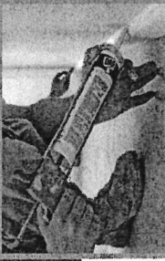
Caulk cracks and spaces
